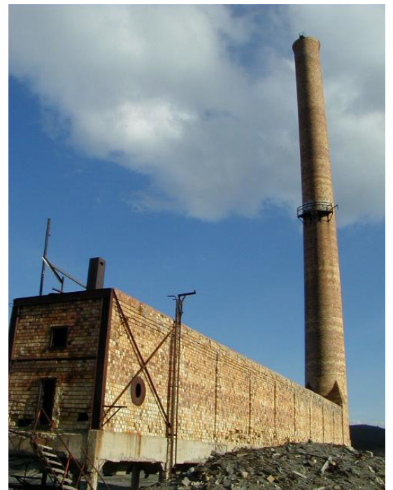
The Humboldt Smelter stack structure.
