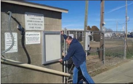
Building Official, Don Roberts installing Bulletin Board
